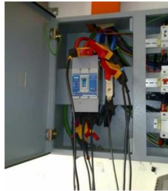
Fig 2: The clamp connection for each phase
