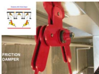
Using rotational friction dampers in retrofiting
